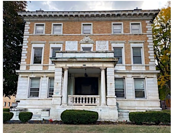
Front elevation of the Rectory.
