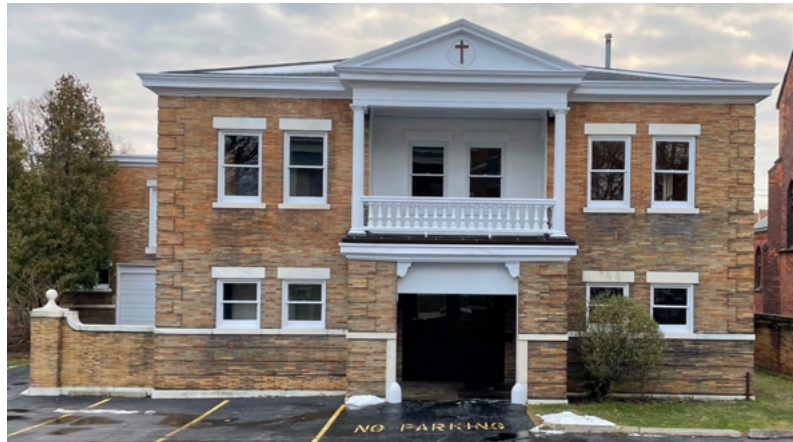
Front elevation of Carriage House.
