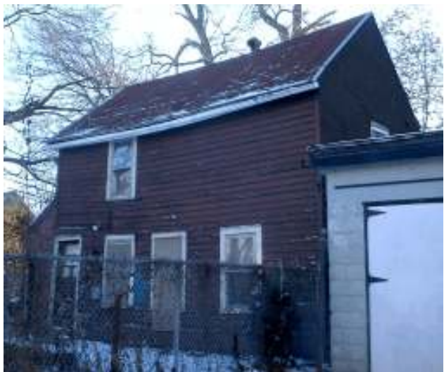
299 Pennsylvania Street, Carpentry Shop in Rear
