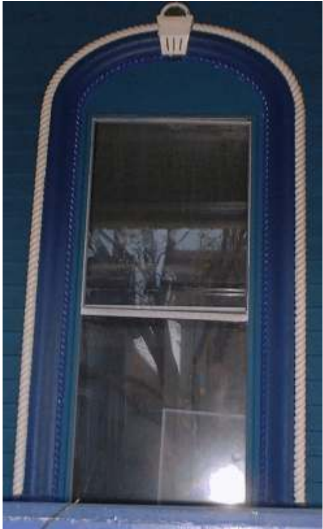
299 Pennsylvania Street, Window Detail
