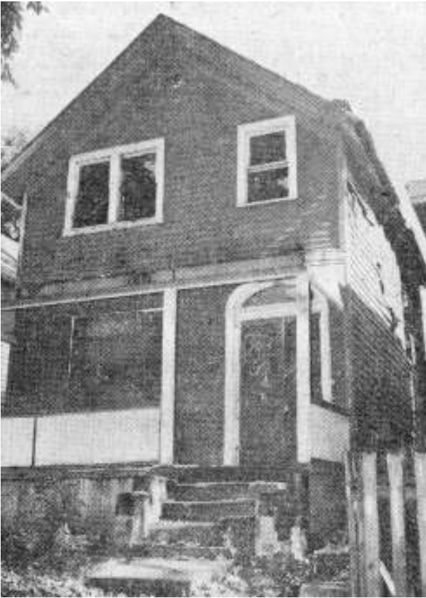
29 Plymouth Avenue, 1967 prior to demolition.
