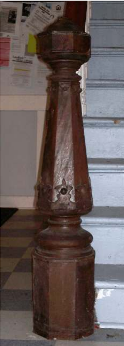
Octagonal newel post found on homes built on Plymouth Ave., from the 1870s.
