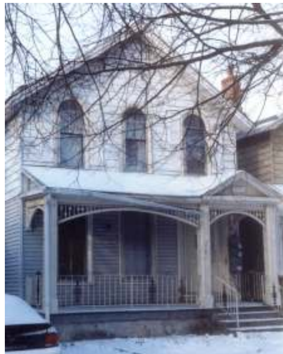
A house that John Cook, Jr. built during the 1870s on Seventh St. that retains its arched windows and porch. This house is very similar to those he built on Plymouth Ave. and to the designs published by S.B. Reed.
