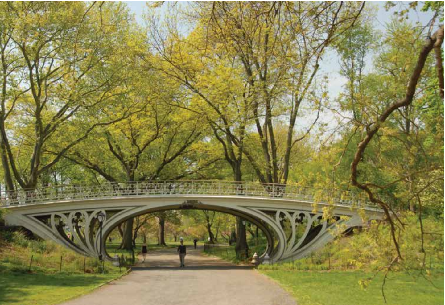
Bridge No. 28 (Gothic Bridge), Central Park. Photograph by Sara Cedar Miller/Central Park Conservancy.
