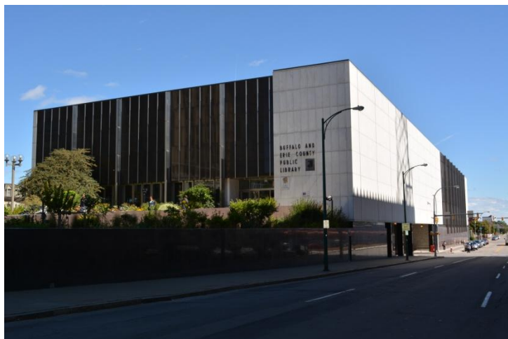
Photograph 4.8. Central Library Branch, Buffalo & Erie County Public Library ( Panamerican 2013 ).
