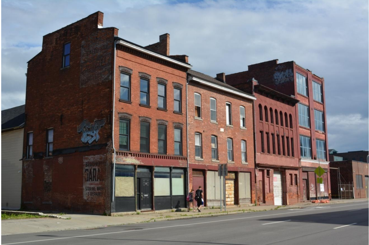
Photograph 4.12. An extant row of mid-to-late nineteenth century commercial buildings at 173-181 Elm Street (Panamerican 20013).
