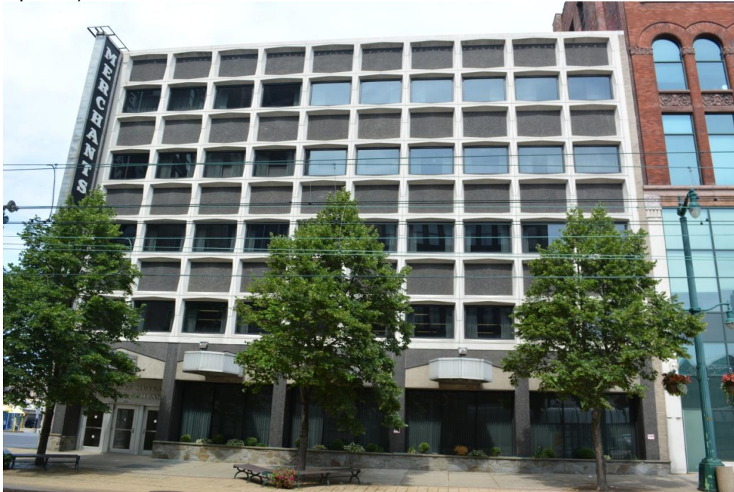
Photograph 4.1. Merchants Mutual Building at 246 Main Street ( Panamerican 2013 ).
