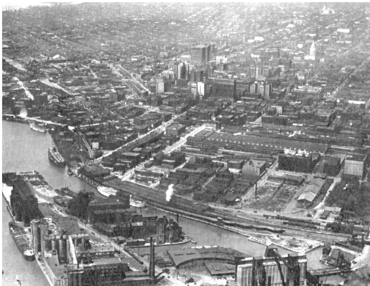
Figure 3.6. The southern portion of the Downtown survey area in 1924. Note: DL&W coal trestle at upper left, the DL&W terminal along the river, and numerous grain elevators on Kelly Island (Ronne & Washburn 1924).
