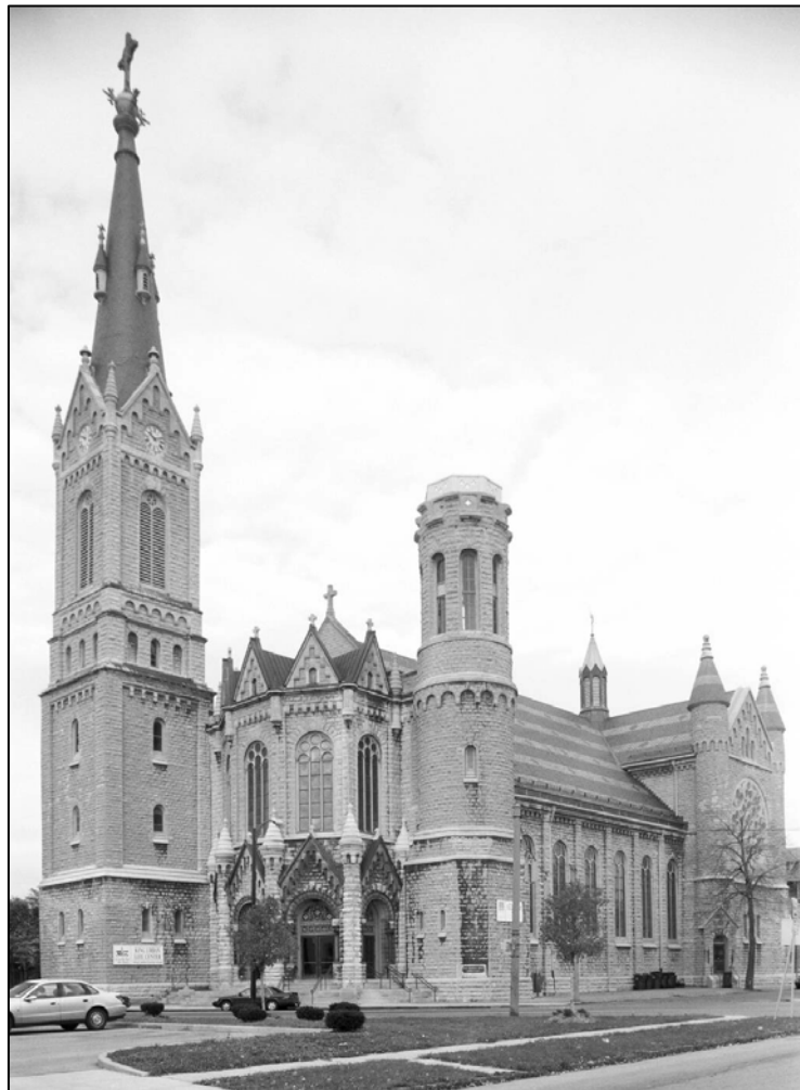
Figure 3.10 St. Mary of Sorrows Church at 935 Genesee Street (1887-1891; Adolphus Druiding, architect. The building is built of local Buffalo Plains blue limestone. The interior was gutted by a fire in 1947, and was reconstructed the following year to the designs of Schmill, Schmill & Hoffmeyer.
