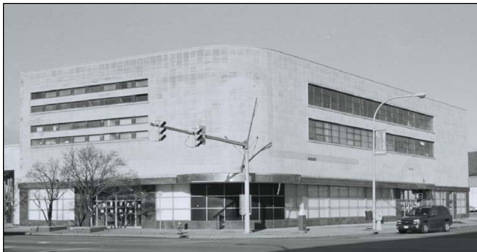
Figure 3.34 Bley & Lyman’s John C. Eckhardt department store (1940) at the northwest corner of Broadway and Fillmore Avenue (950 Broadway). It one of the most significant early Modern buildings surviving in Buffalo.
