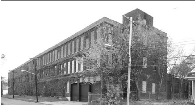
Figure 3.39 Esenwein and Johnson' three-story Duffy Silk Company building at 207 Guilford Street.
