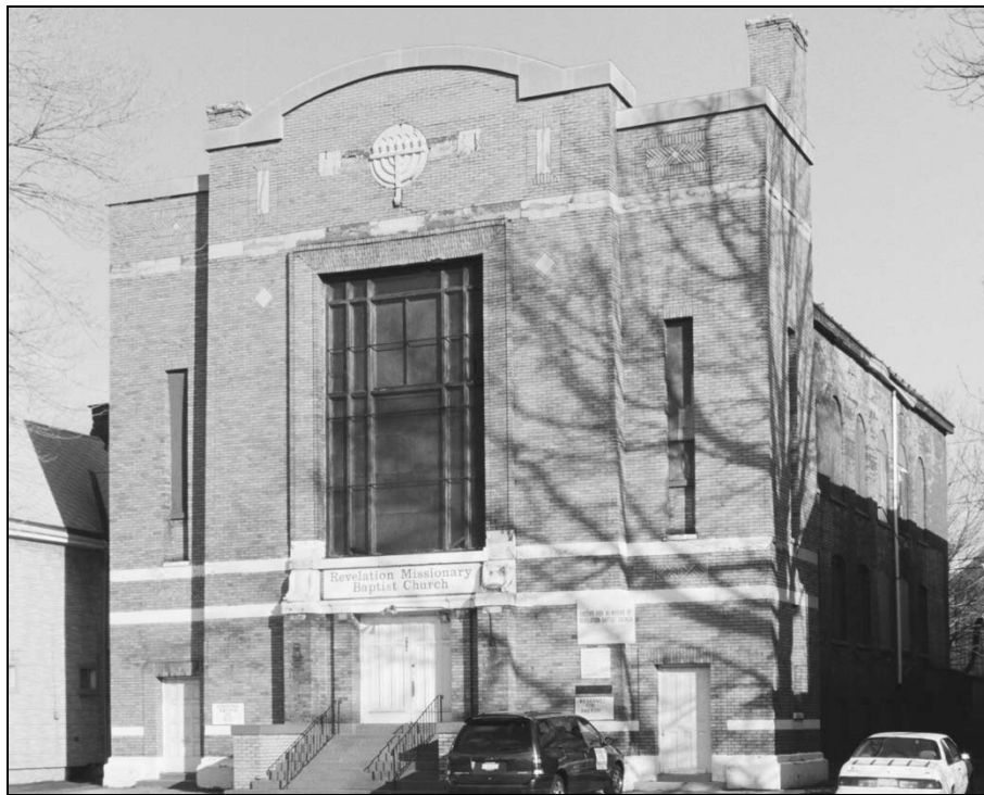
Figure 3.23 Achavas Achim, synagogue at 833 Fillmore Avenue (1912; Henry Osgood Holland).
