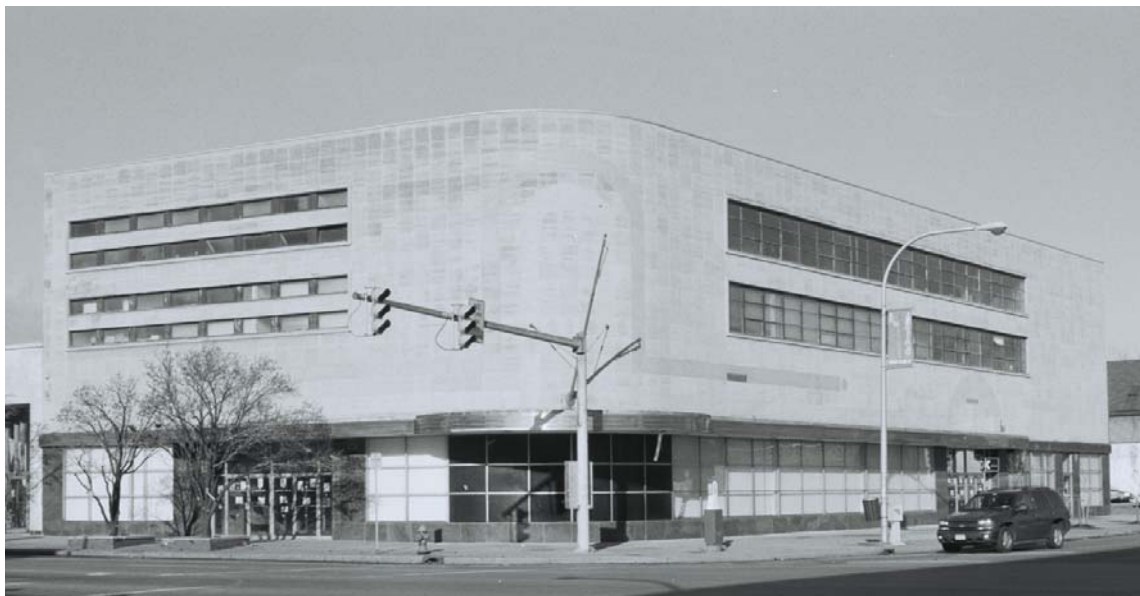
PHOTOGRAPH: (Broadway-Fillmore R-5; N-10)
