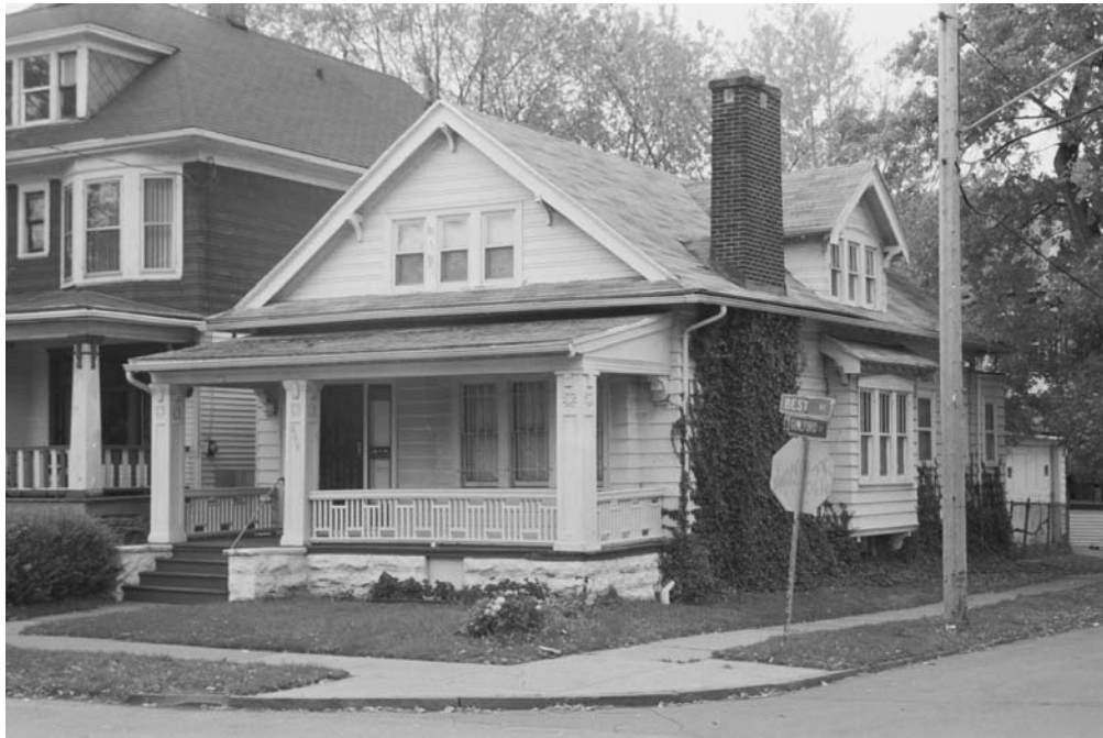
PHOTOGRAPH: (Broadway-Fillmore R-1; N-2)
