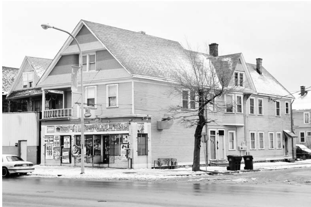
PHOTOGRAPH: (Broadway-Fillmore R-14; N-5)
