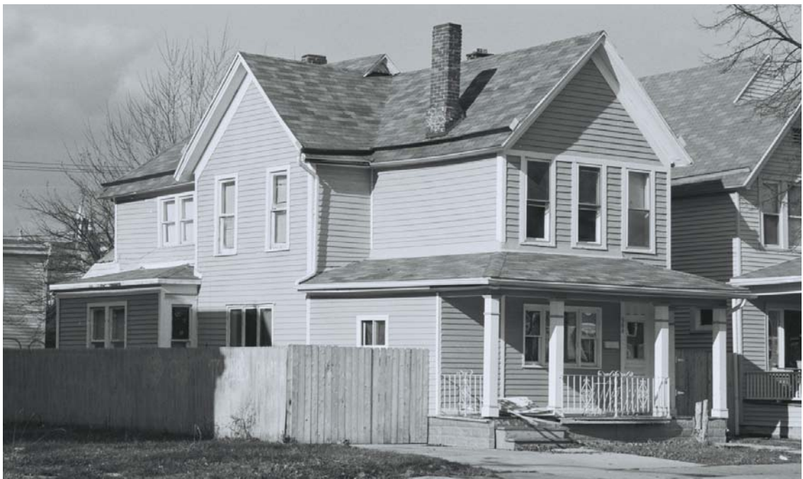
PHOTOGRAPH: (Broadway-Fillmore R-5; N-22)
