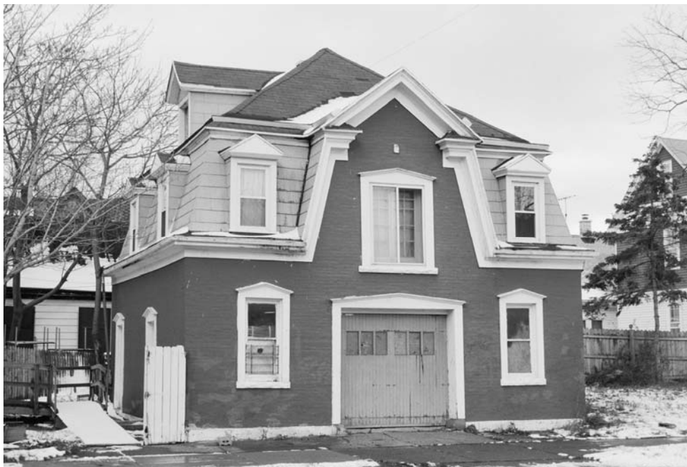
PHOTOGRAPH: (Broadway-Fillmore R-15; N-1)
