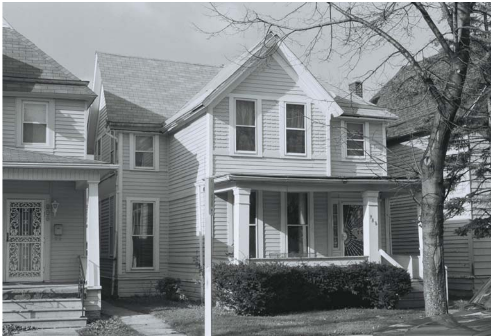
PHOTOGRAPH: (Broadway-Fillmore R-5; N-23)
