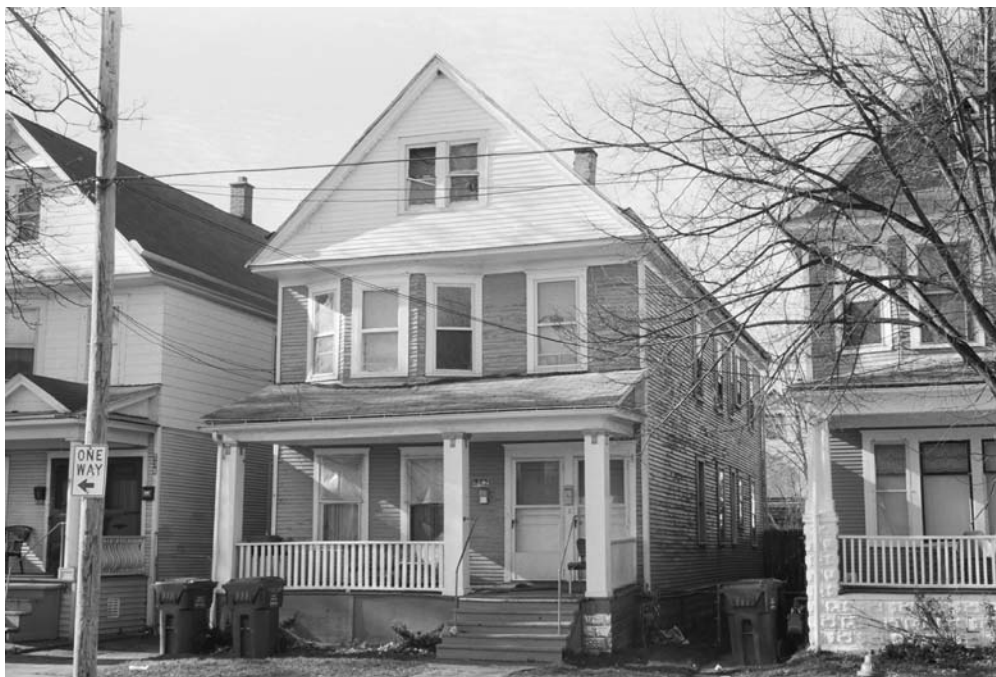
PHOTOGRAPH: (Broadway-Fillmore R-10; N-13)
