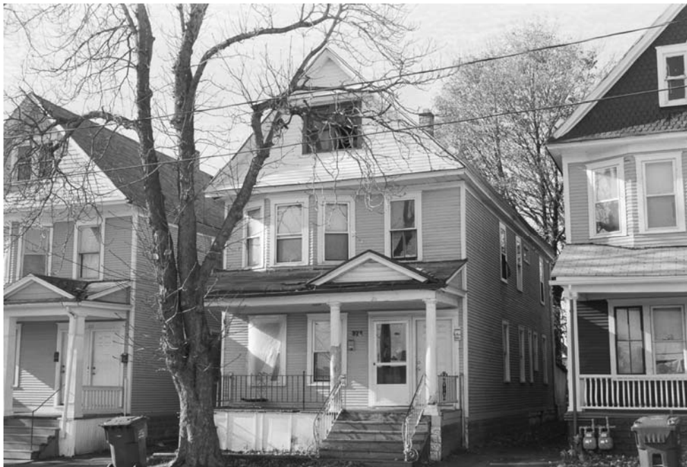
PHOTOGRAPH: (Broadway-Fillmore R-10; N-17)
