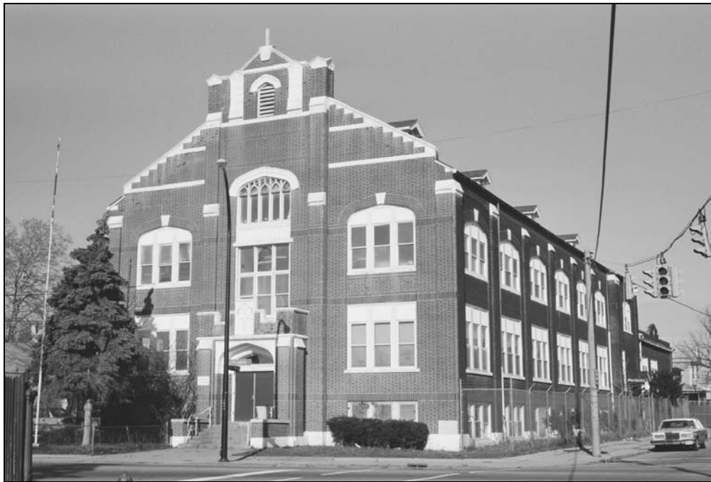
Figure 3.19 Queen of the Most Holy Rosary Church at 1040 Sycamore Street (1916; Wladyslaw H. Zawadzki, architect).
