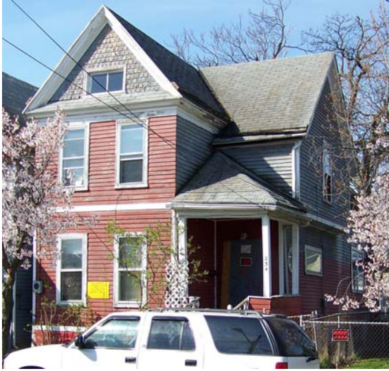
Photo 5.12 234 Thompson Street A good example of the gabled ell type Folk Victorian house with decorative shingles in the front gable.
