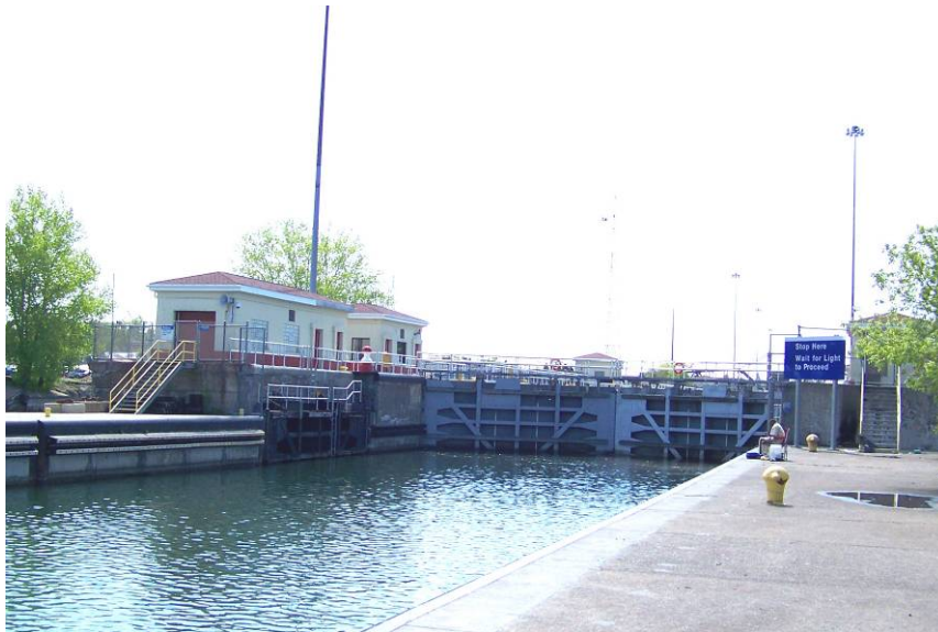
Photo 5.22 Black Rock Canal and Lock
