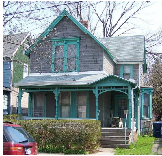
Photo 5.13 301 Dearborn Street Despite asbestos sheathing, this L-plan house retains an excellent Victorian porch and intact window surround.
