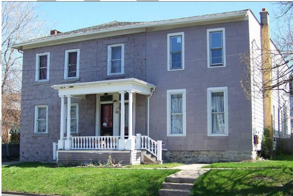
Figure C-2: The Samuel Howell House, 189-191 Dearborn Street (ca. 1830, addition ca. 1870s) An excellent example of a stone-constructed residential building of the Federal Style.
