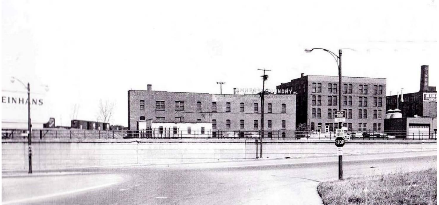
Figure B-19: Looking north on Tonawanda Street at Amherst Street (May 2, 1963)
