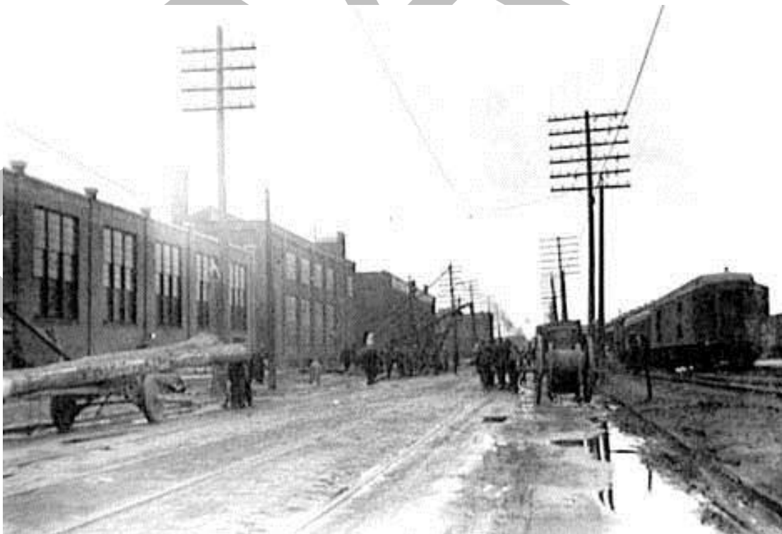
Figure B-46: Looking south on Tonawanda Street, Pratt & Letchworth factory at left (March 16, 1923)
