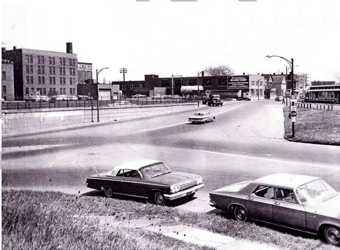
Figure B-20: Looking east down Amherst Street at Tonawanda Street (May 2, 1963)
