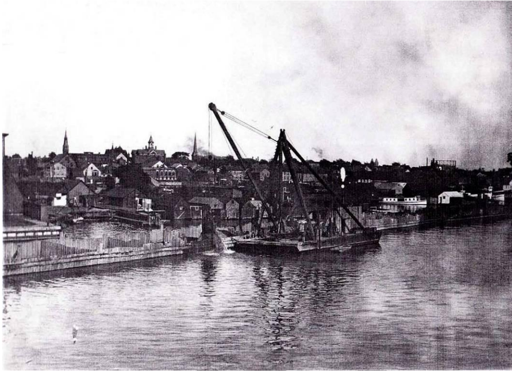
Figure B-11: Black Rock Harbor Construction and Cofferdam (1908-09)
