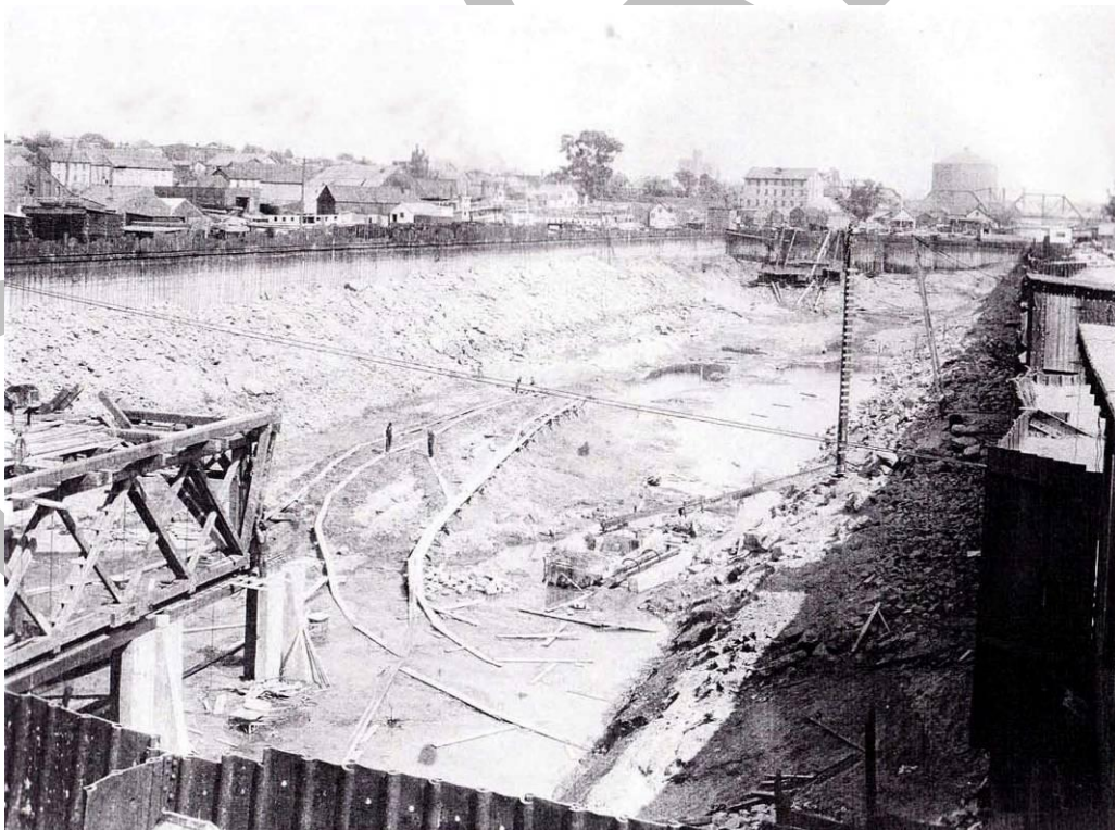
Figure B-10: Black Rock Harbor Construction and Cofferdam (1908-09)
