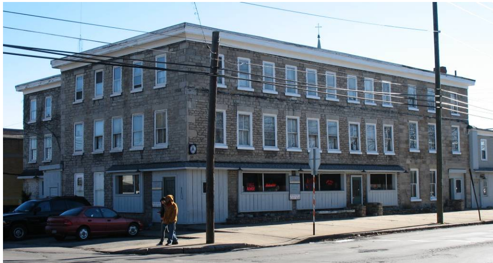
Photo 5.36 58 North Transit Street The Niagara Hotel is a rare, excellent large-scale example of stone construction. Historically the building had a large 2-story porch with columns, and the ground floor has been altered, but otherwise the exterior is remarkably intact from its ca. 1850s appearance.
