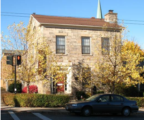
Photo 5.34 32 Cottage Street The NR-listed Bacon-Merchant-Moss House (ca. 1832) is a residential example which uses Medina sandstone in its construction.
