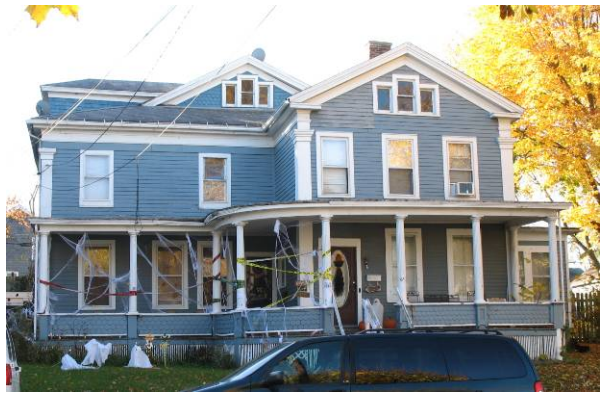
Photo 5.3 64-66 Genesee Street A gable front and wing example, this house features corner pilasters and a wide entablature molding at the eaves. Note the later alterations including a porch and dormer.
