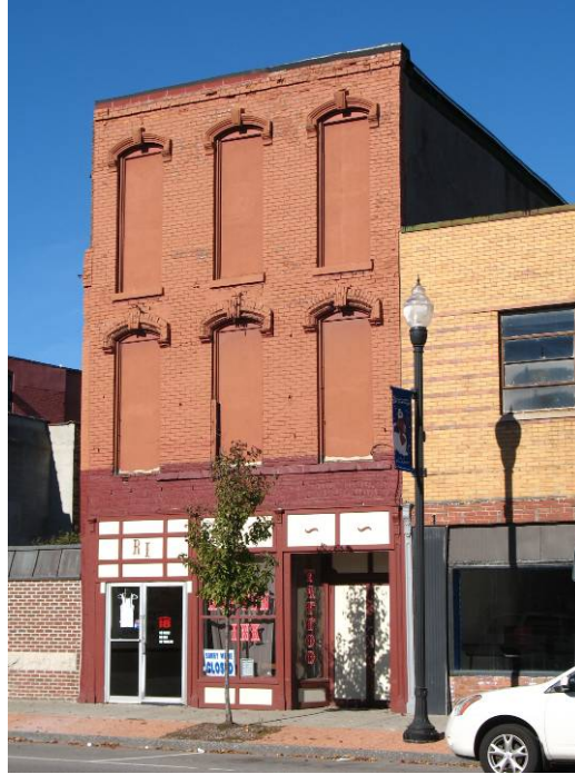
Photo 5.8 17 West Main Street Although the windows are boarded, the upper floors of this building retain their signature Italianate hood molds.
