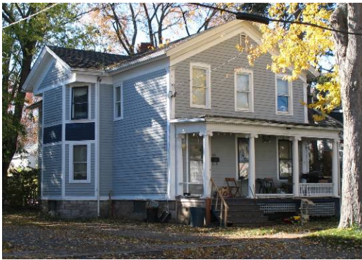
Photo 5.2 188 Genesee Street A front-gabled example with a full-width porch with Ionic columns, pedimented window hoods and entablature molding with dentils. Later cross-gabled wing.
