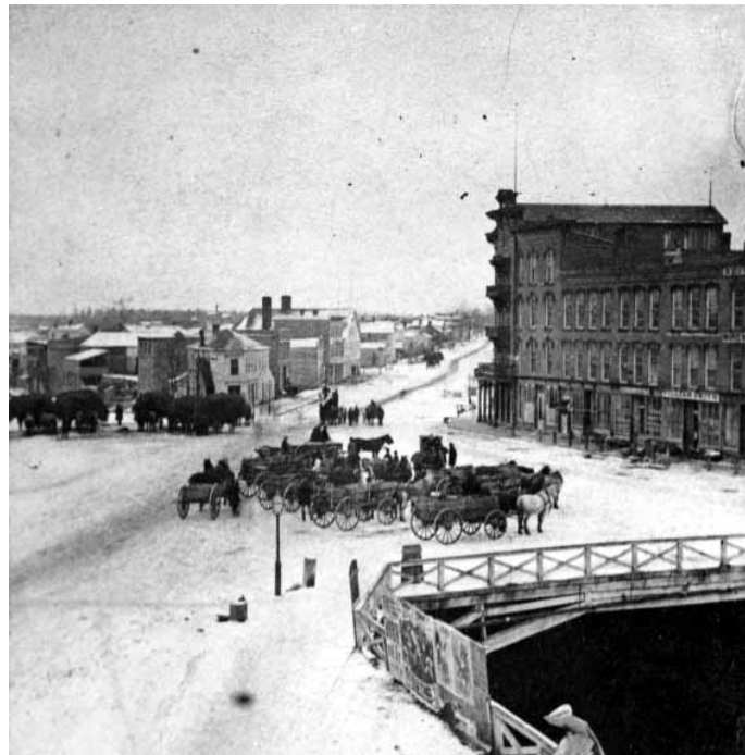
Figure 4.19 Lockport's "Big Bridge" (1875) 80
