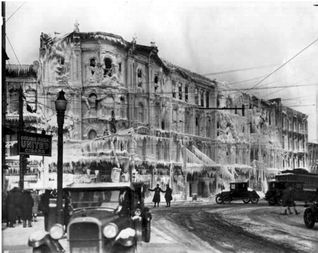
Figure 4.30 The devastated Hodge Opera House in 1928 following the fire. 104
