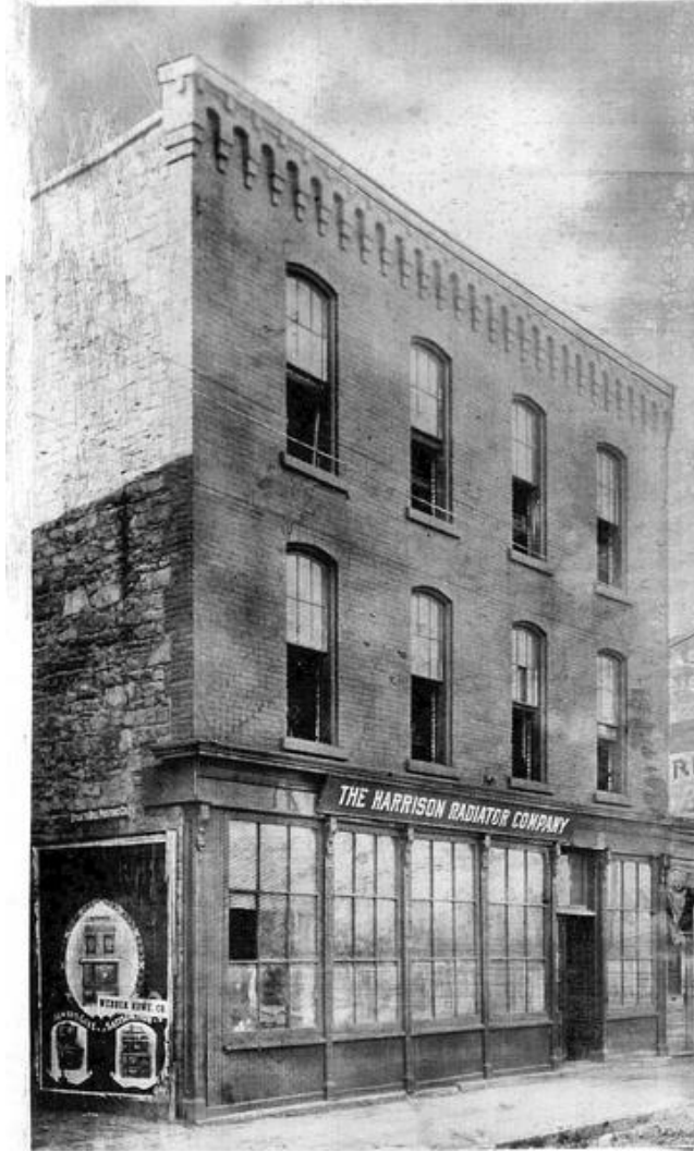
Figure 4.34 The Harrison Radiator Company Building, Elm Street (undated, ca. 1910s) 108
