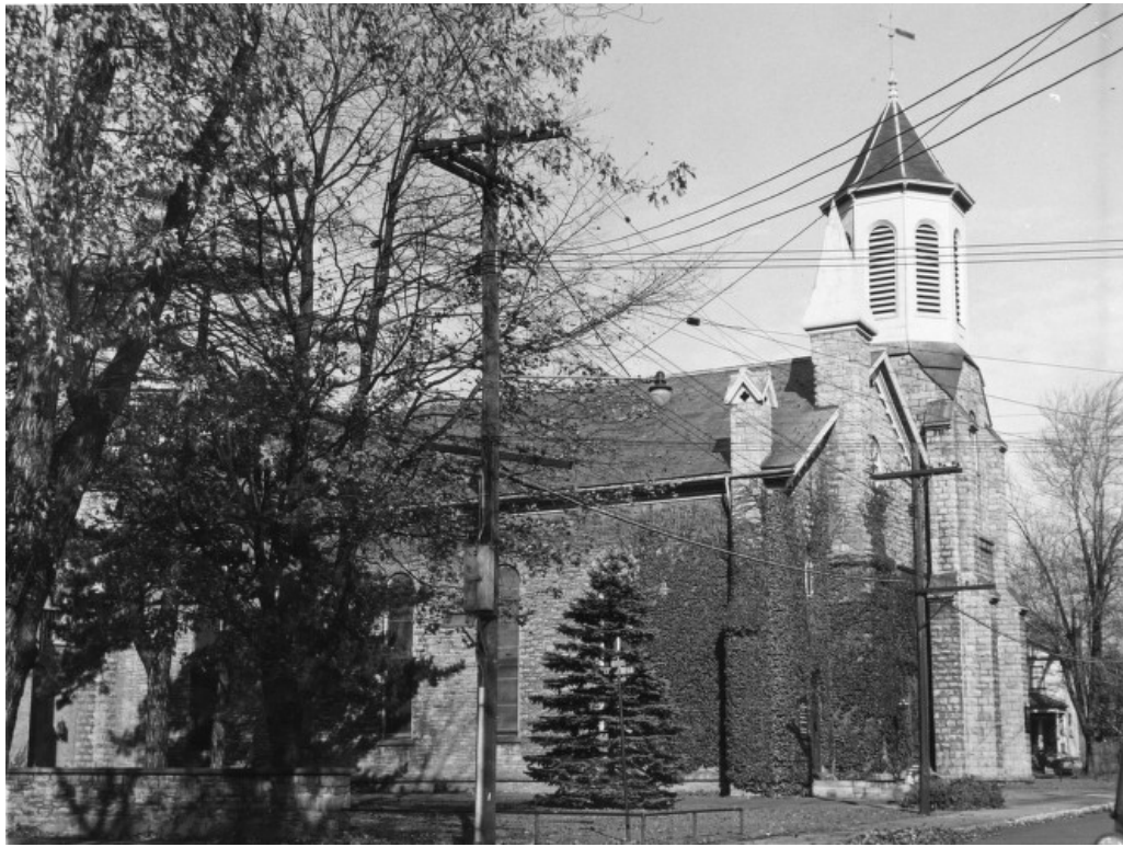
Figure 4.38 First Presbyterian Church, Lockport (Oct, 26, 1946) 116 Note the changes to the steeple and the removal of the spire.
