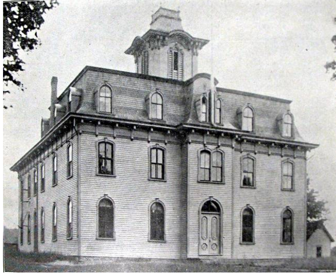
Figure 22 Sherman's old school house, built 1869 (demolished)
