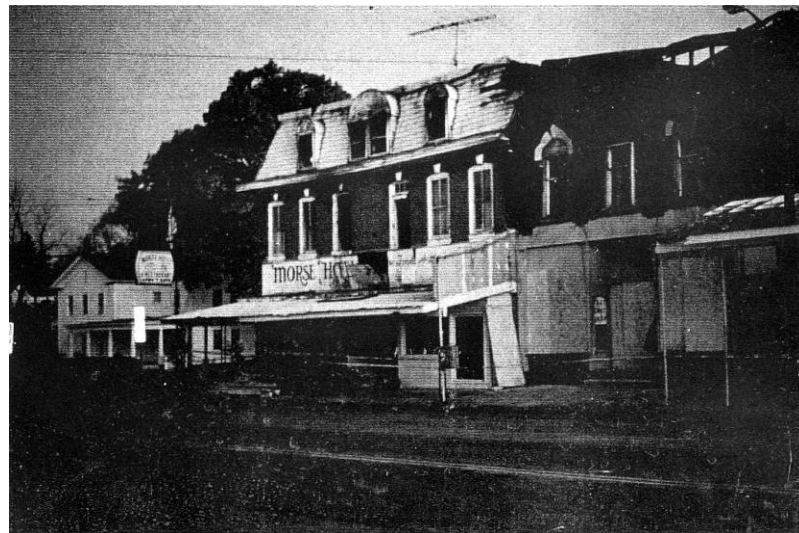
Figure 29 The Morse Hotel destroyed by fire, 1991
