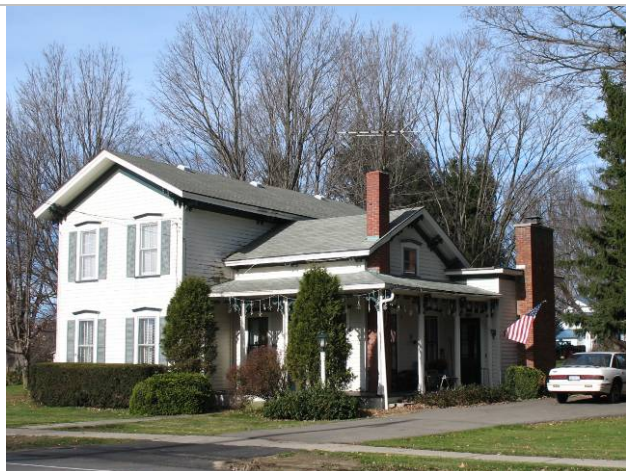
The Hazlet House 185 Park Street Ca. 1870
