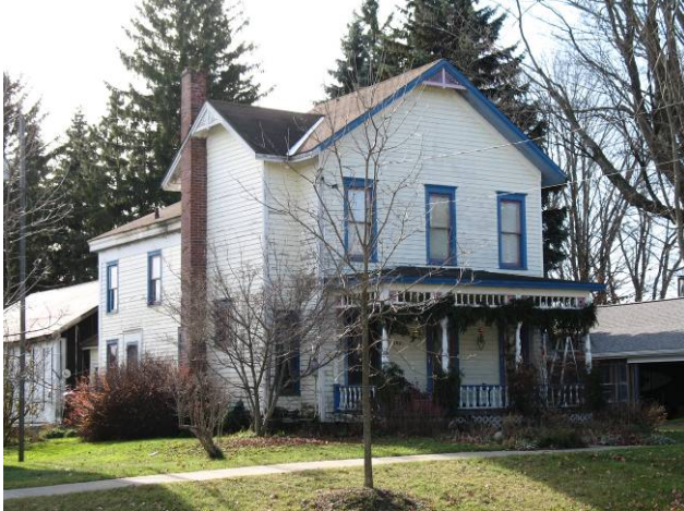
The Former Presbyterian Parsonage 142 Main Street Ca. 1855; altered 1890
