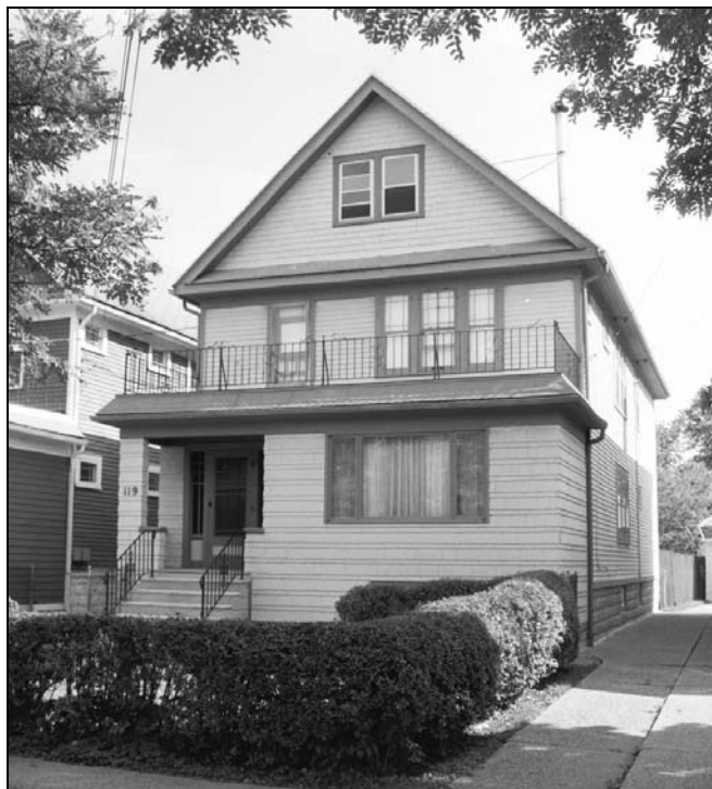
Figure 3-12. Two-family house (‘flats’) at 119 Folger Street (1924; James McNaught, builder)
