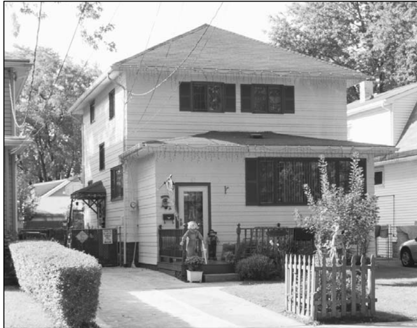
Figure 3-4. Single-family house at 69 Crystal Avenue (1926) built by Lodge Realty Corp.
