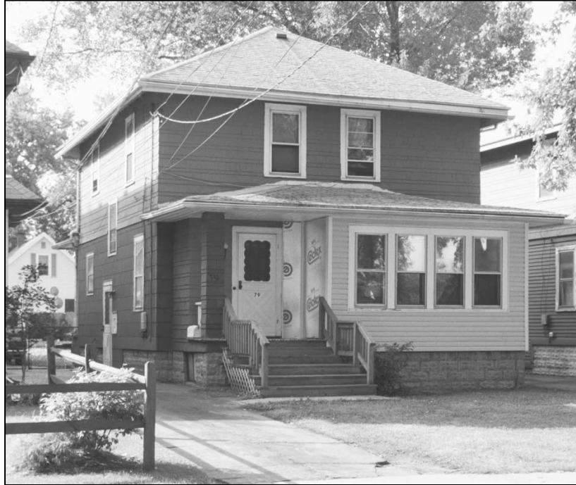
Figure 3-6. Single-family house at 79 Crystal Avenue (1926) built by Lodge Realty Corp.
