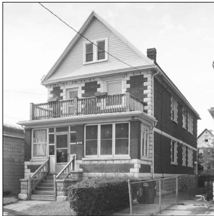
Figure 3-7. John Jepson's single-family house at 102 Macamley Street (1911)
