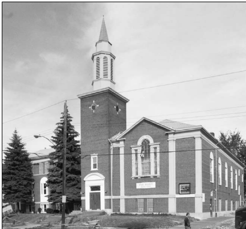
Figure 3-14. South Park Baptist Church (1925) at 187 South Side Parkway Designed by North, Shelgren & Swift, architects
