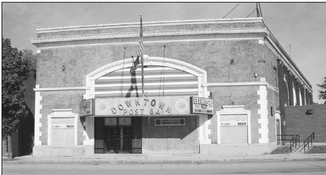
Figure 3-16. Henry L. Spann's South Park Theatre (1919) 1770 South Park Avenue
